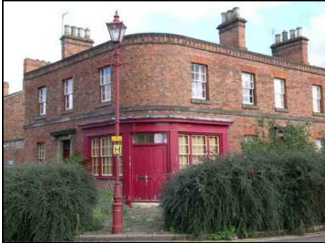
Examples of Tripartite vertical sliding sash windows
