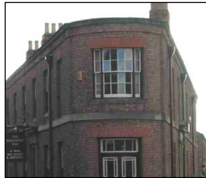
Examples of Tripartite vertical sliding sash windows
