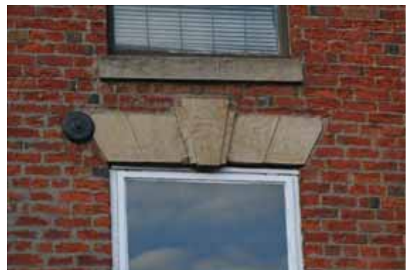
Pink gritstone from the Matlock area of Derbyshire was adopted for the whole building at the former Municipal Technical College (left). Wedge lintels carved from buff gritstone quarried from the Melbourne area at Green Lane (right)
