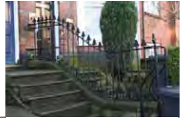
Cast iron round-section railings with spear-headed finials at Wilson Street (above & below) and Macklin Street (left)
