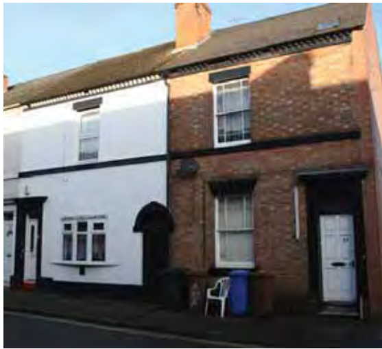
Left - original Flemish bond brickwork covered with render, wedge stone lintel removed, window re-formed & sash windows replaced (Crompton Street) Right - concrete roof tiles replace Welsh slate or clay tiles (Green Lane)
