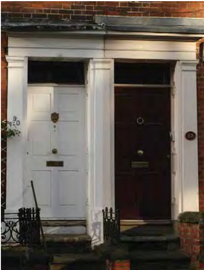
Right - stone classical doorcase with pilasters, entablature, egg-and-dart moulding & ornamental panelled door
