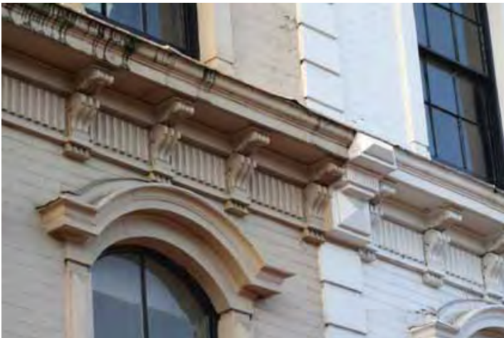
Left - stone rusticated quoins and pilasters, stone cornice with console brackets and frieze with an interpretation of classical triglyphs (46-52 St. Peters St)
