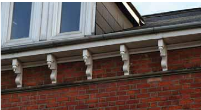
Right - in the second half of the 19th century eaves were often highly decorative, built using moulded bricks or terracotta to create complicated corbelled details. The elements together mimic a classical cornice (32-34 St. Peters Churchyard, 52 & 91 Green Lane).
