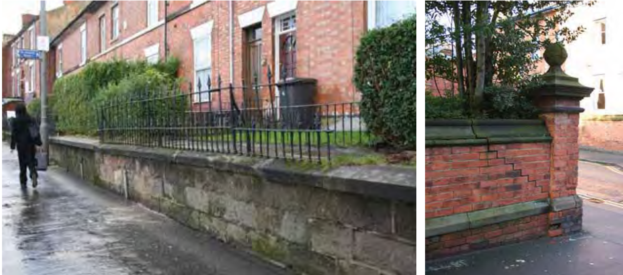
Ashlar stone wall with decorative cast iron railings at Victoria Terrace (left) & brick wall with moulded stone capping & corner pier at Stuart Terrace, Green Lane (right)
