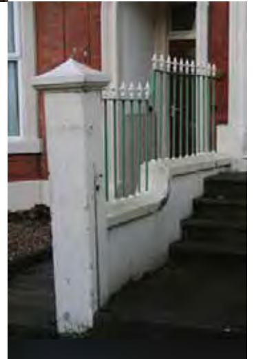
Cast iron round-section railings with spear-headed finials at Wilson Street (above & below) and Macklin Street (left)
