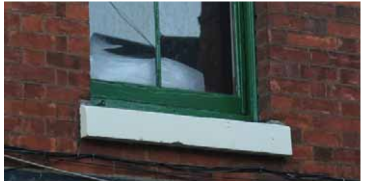
Cills - most of the cills within the area are stone & chamfered with a weathering (above). Many stone cills run into a stone band (right)
