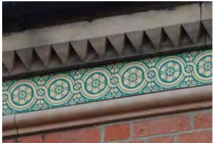
Right - elaborate moulded stone and encaustic tiled eaves at 125 Green Lane
