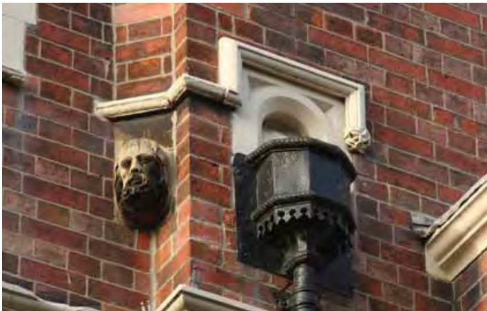
Above - carved stone head of a medieval figure forms a decorative corbel at 110 Green Lane. The decoration extends to the lead rainwater hopper, which is made with gothic style fleur-de-lys and rope edging
