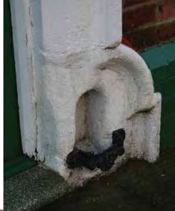
Above - cast iron boot scraper, set in stone, at Crompton Street, once a common detail outside domestic buildings
