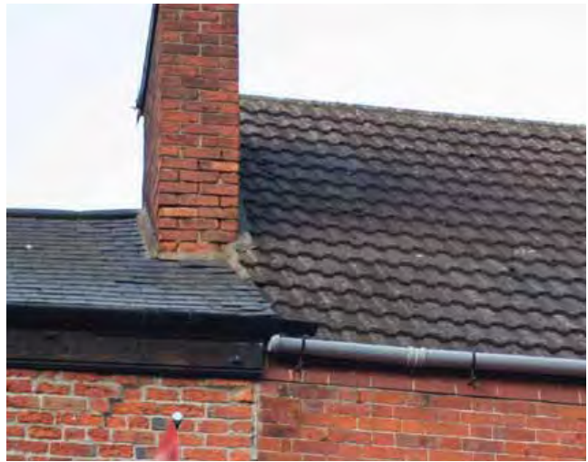
Left - original Flemish bond brickwork covered with render, wedge stone lintel removed, window re-formed & sash windows replaced (Crompton Street) Right - concrete roof tiles replace Welsh slate or clay tiles (Green Lane)
