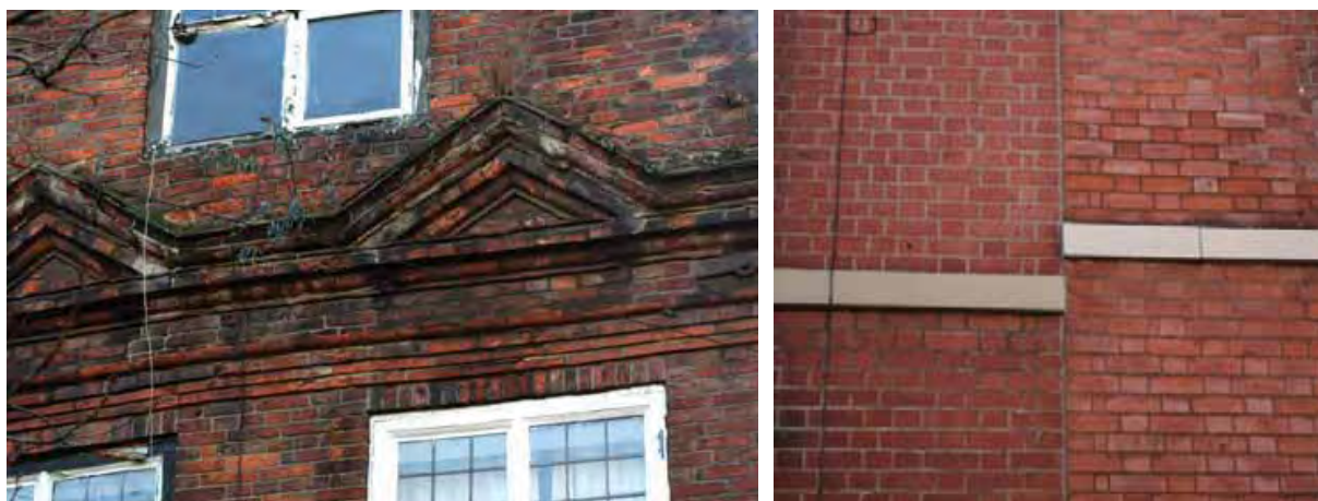
Left - the former Green Man Inn - 17th century moulded brickwork. Right - 19th century Flemish bond brickwork at Crompton Street
