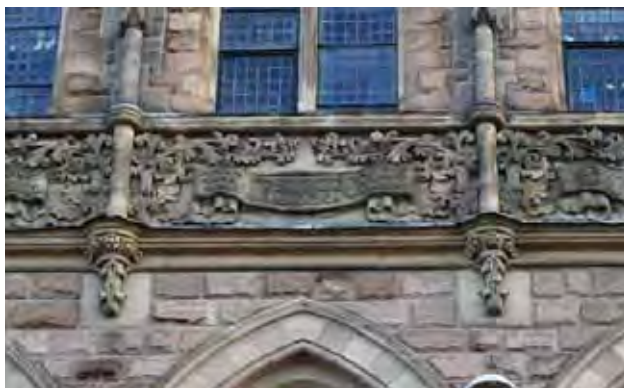
Pink gritstone from the Matlock area of Derbyshire was adopted for the whole building at the former Municipal Technical College (left). Wedge lintels carved from buff gritstone quarried from the Melbourne area at Green Lane (right)
