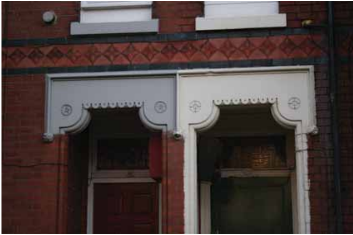
Above - door lintels of stone with carved details to the soffit (58-59 Wilson Street). The shape is based on a shouldered arch, a detail found in medieval buildings
