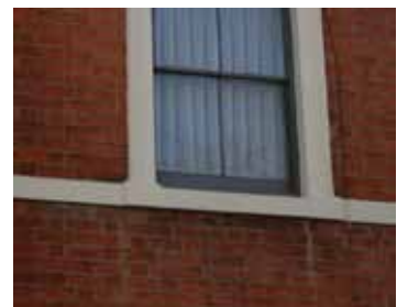
Cills - most of the cills within the area are stone & chamfered with a weathering (above). Many stone cills run into a stone band (right)
