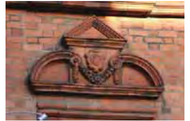
Right - lintel with moulded terracotta pediment & swags, dating from c1890 at No. 54 St. Peters St
