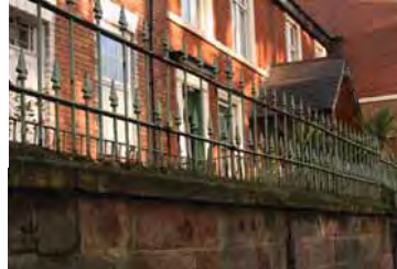
Cast iron round-section railings with spear-headed finials at Wilson Street (above & below) and Macklin Street (left)
