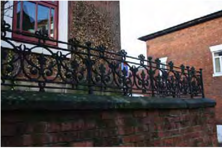
Shallow, decorative cast iron panel railings, fixed to a moulded stone capping & brick wall at 88-90 Green Lane (above)
