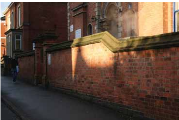
Red brick walls with deep, moulded stone coping at the Beaconsfield Club, Wilson Street (above)
