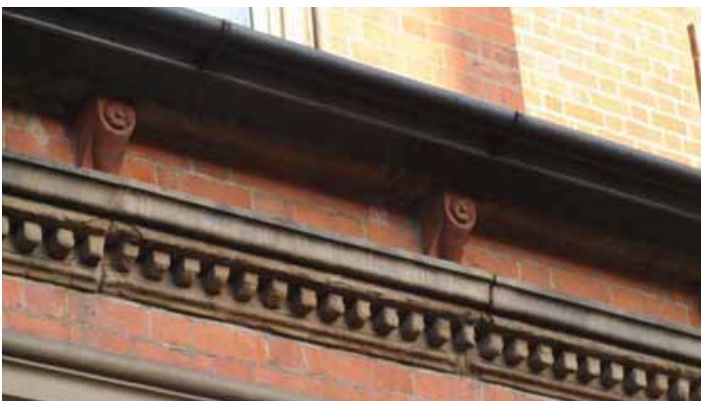
Below - stone cornice with carved dentilled moulding and terracotta rosettes above, an unusual combination at 10 Wilson Street
