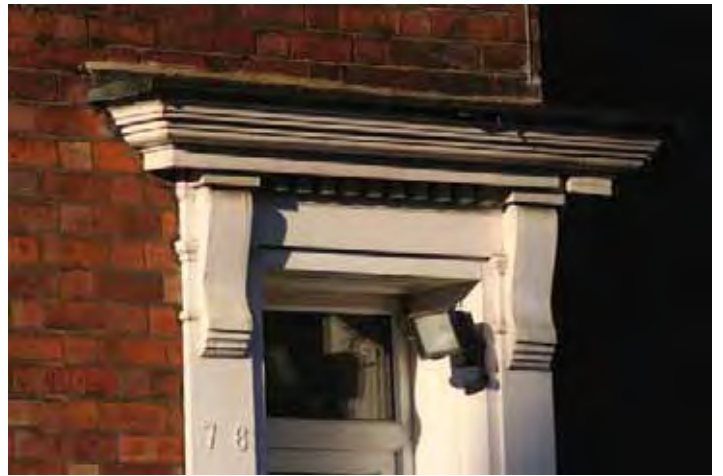
Left & above - simple timber doorcases with panelled linings, fanlights, pilasters & cornice, all late Georgian, classically inspired elements
