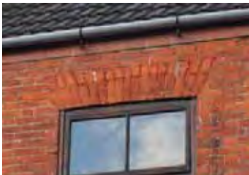
Rubbed & gauged brick lintel (above left) at 32 Green Lane, a detail found in 18th century buildings. The joints were sandwiched together with lime putty. Additional incised lines were applied to simulate lime putty joints & create a regular, refined appearance
