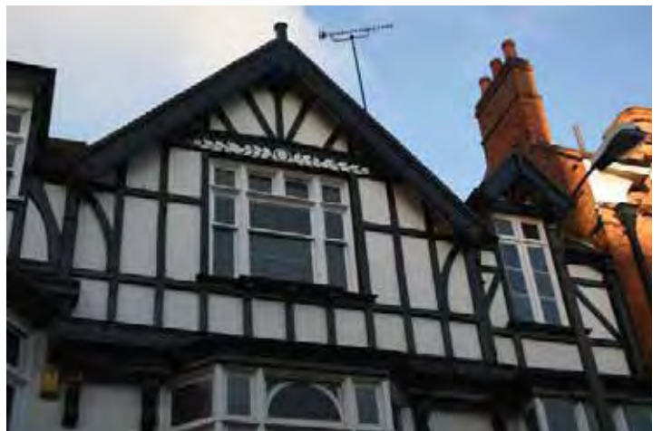
Timber-frame - jettied walls of timber-frame with herringbone brick & plaster panels & ornamental bargeboards (8 St. Peters Churchyard). The Arts & Crafts movement revived some early traditions
