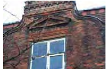
Right - lintel of moulded, rubbed bricks with triangular pediment dating from circa 1671 (the former Green Man Inn)
