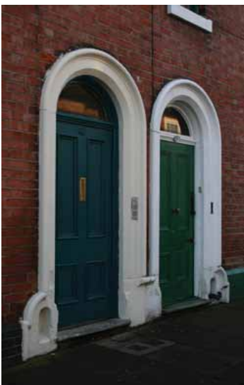
Left - round-arched stone architraves with roll-mouldings & integral bootscrapers, semi-circular fanlights and four-panel doors, with bolection mouldings - 27-28 Crompton Street
