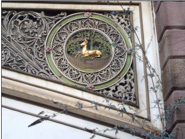
Delicate cast iron ornament in the spandrel of the Friar Gate Bridge (1876)
