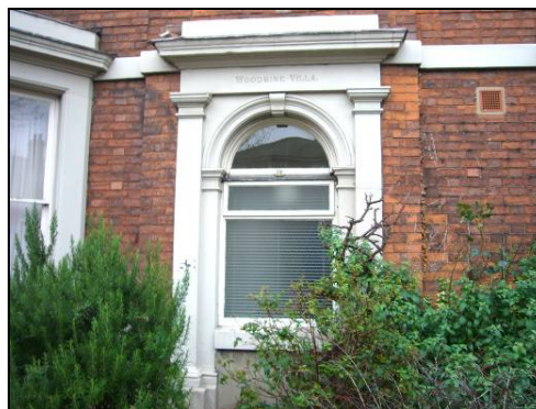
Negatives: parapet in need of repair at nos. 30/31 Friar Gate (left); insensitively blocked doorway in Ashbourne Road (right).
