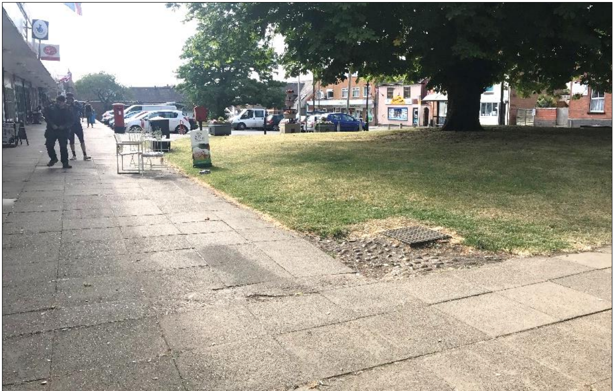
Figure 3.4 Broken footway within the shopping area
