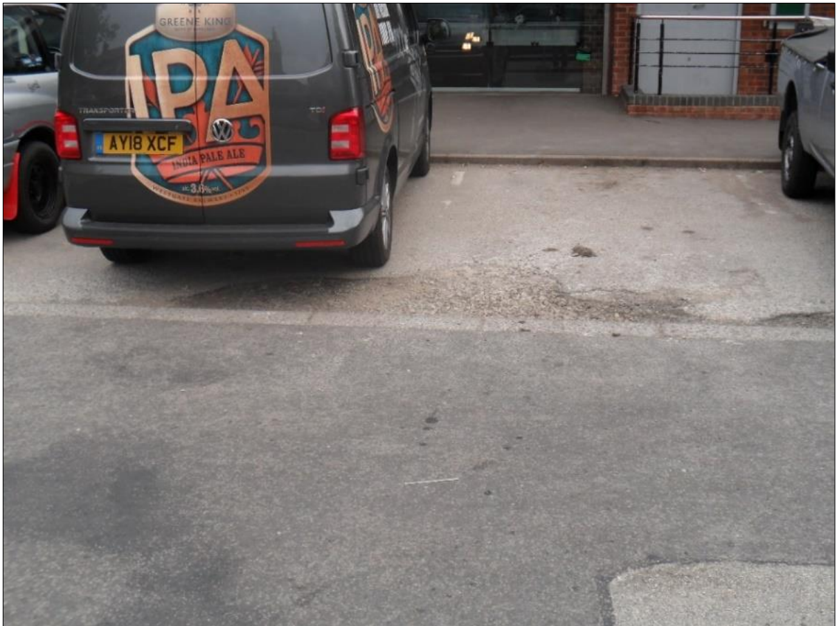
Figure 6.2 Uneven surface in car park on Uttoxeter Road
