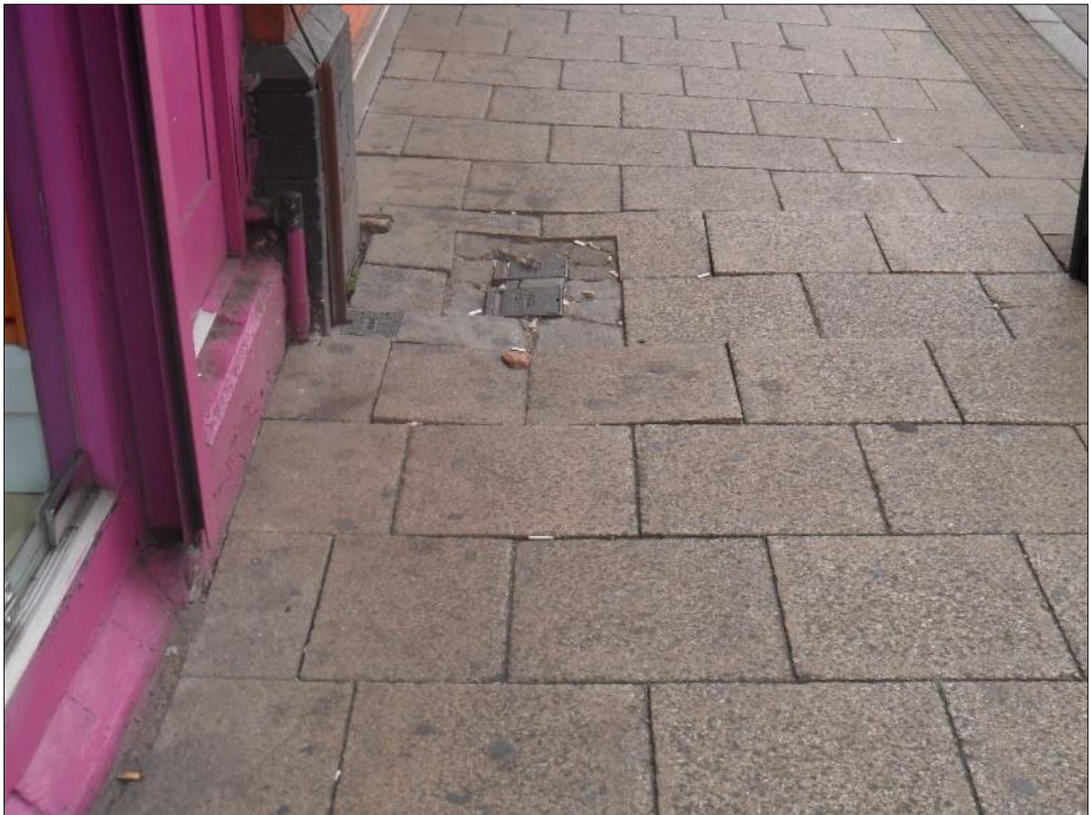
Figure 6.1 Broken and uneven footway surface within retail district.
