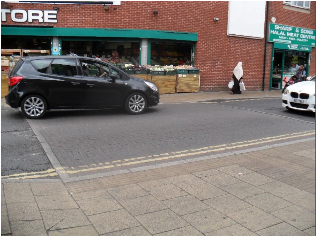
Figure 3.6 Raised Speed Table Crossing on Pear Tree Road
