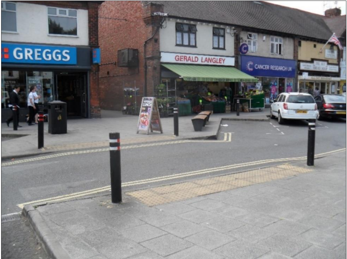
Figure 3.5 Raised Speed Table within the Shopping Area - Osmaston Rd
