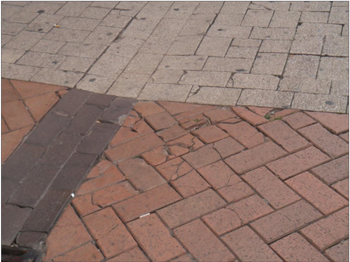
Figure 3.17 Cracked footway in Pedestrianised Zone - Sadler Gate - Cathedral Quarter
