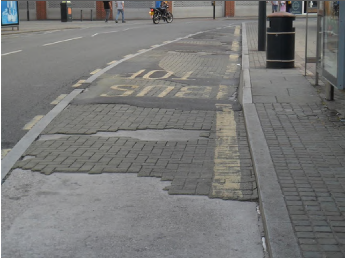
Figure 4.6 Broken & Uneven Bus Layby Surface on Albert Street - St Peters Quarter
