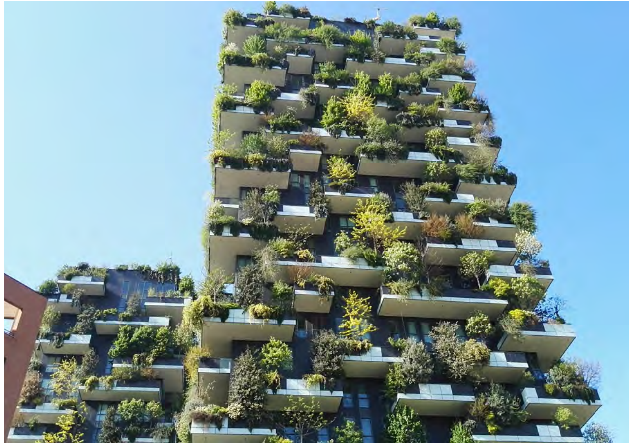
Figure 3.44: Bosco Verticale (“Vertical Forest”) In Milan is a pioneering example of vertical greening on a tall building
