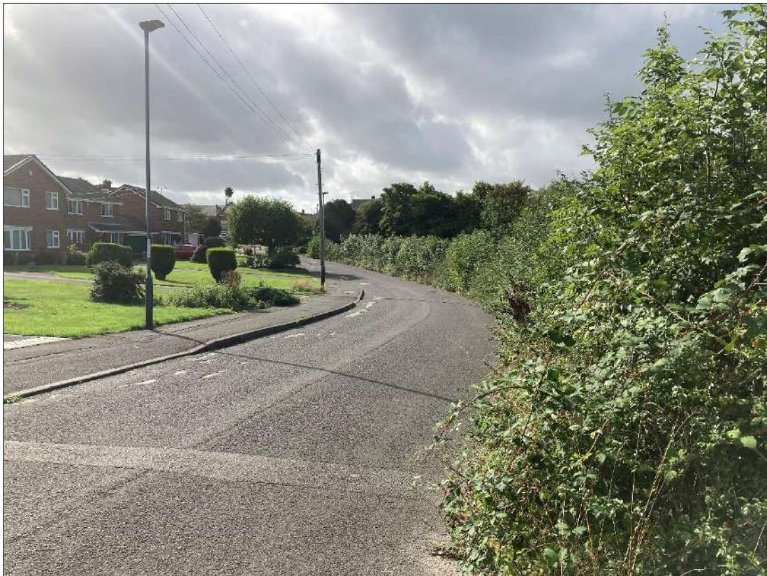
Figure 1.4: Looking south on Royal Hill Road towards Low Point at Site Access
