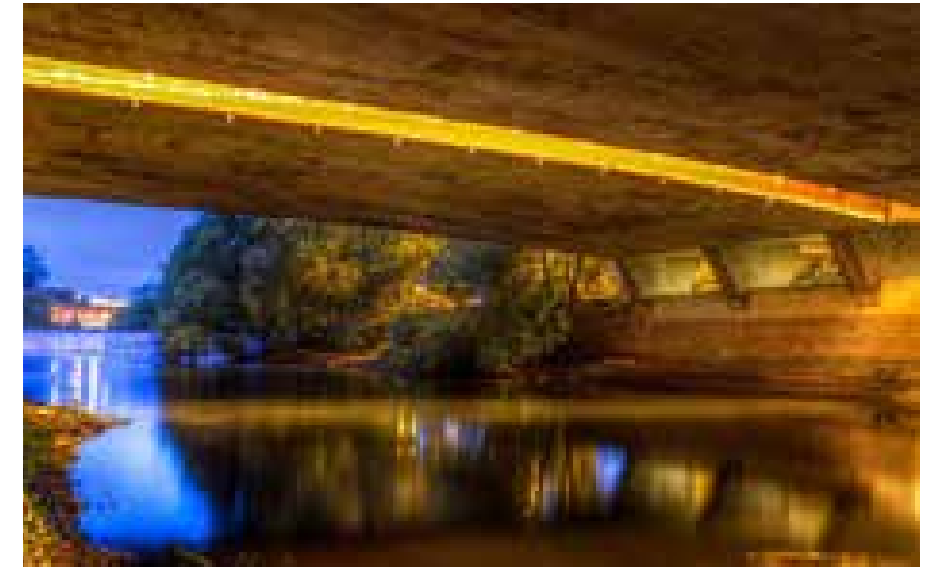
Tunnel Vision Project
