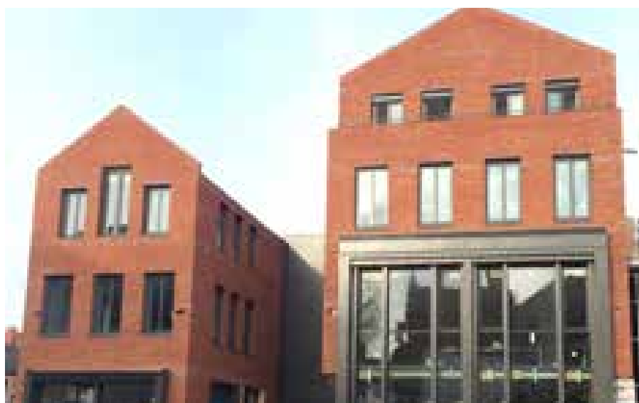
Sadler Bridge Studios
