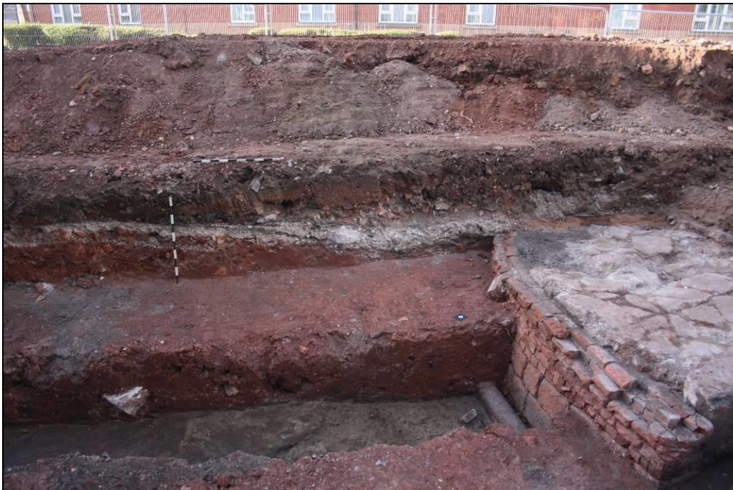
Figure 3. East facing section of Trench 801 showing location of concrete and 33kVA cables
