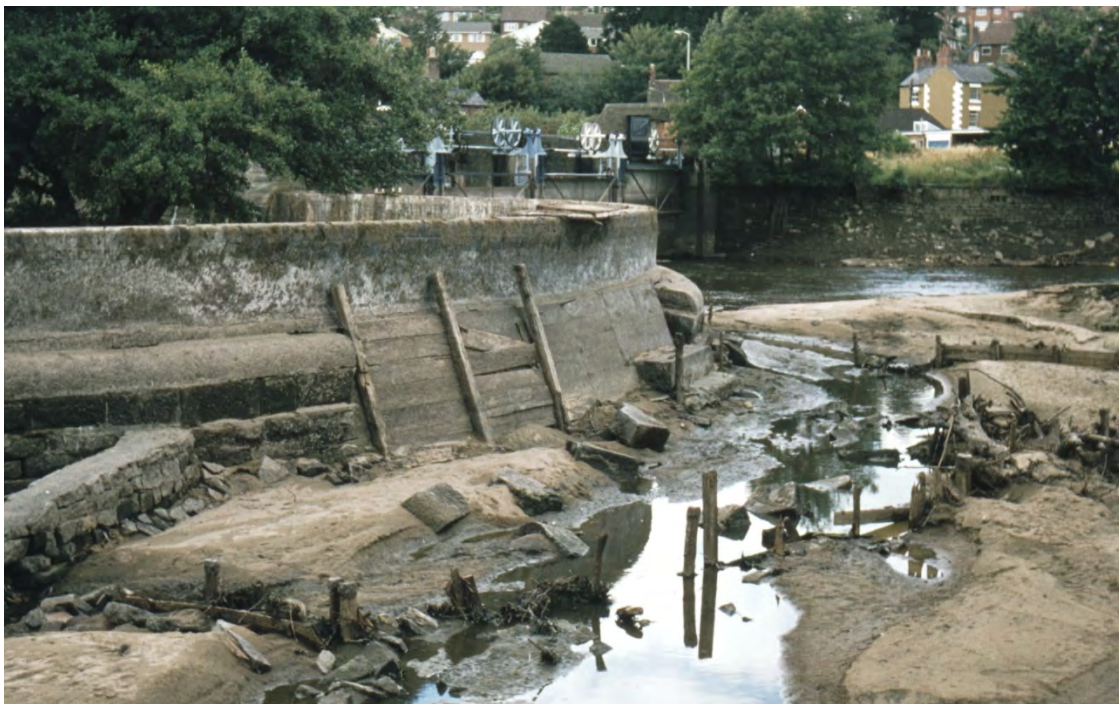
Fig.34 Remains of coffer dam with timbers embedded in the river bed above Belper Horseshoe Weir in 1976 (© Courtesy of Belper Historical Society – BHS02569)
