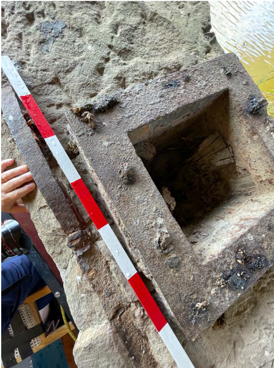
Fig.38 Cast-iron square collar with inset casting surrounding a timber post (parts of which are visible) let into the upper face of the stone pier and bolted to the upper face with 4 corroded bolts. The outer edge of the collar measures approximately 500 x 500mm. Off-set is a wrought-iron cramp 350mm long inset into the stone at the joint between two large masonry blocks and another channel cut for a wrought iron cramp which is missing. The stone appear to have delaminated at the outer edge, where it is fractured and a weak spot – 8.8.2025.
