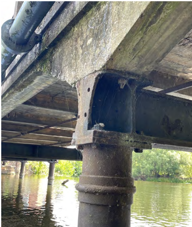
Fig.41 Tapered end of cast-iron beam, with four holes for dowels. The end cap is missing to this beam - 8.8.2025.
