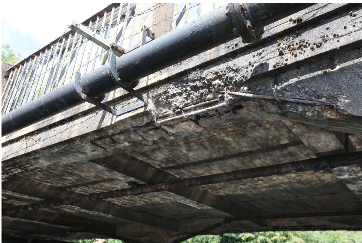
Fig.28 View of downstream face with corroded rebar and spalled concrete, sewer pipe to the side and gas pipe to the soffit (8.8.25)
