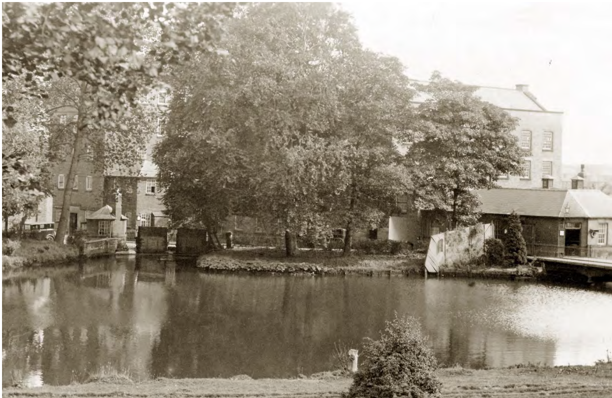
Fig. 10 View of the left bank upstream of the bridge ca. 1930, The water level is high, where it is impounded by the sluices of the weir and this shows the clear relationship between this level and the paired sluices which are visible in this image as two large timber 'walls' adjacent to the watch house, which are in their raised 'operational' position. High railings set between the watch house and the sluices can be seen. The left bank is vegetated, with some signs of a part-timber revetment by this date. We can date the view by the presence of two cars. This glimpse of the bridge suggests an almost completely flat bridge deck and shallow arches springing from the cast-iron 'end caps', one of which is visible, and a slim deck oversailing them and carrying the railings. (Photograph courtesy of Adrian Farmer).
