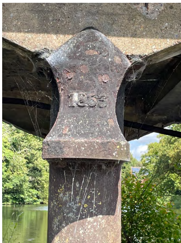
Figs.43 & 44 End caps with visible dowels to upper face (left – plain, right – with 1853 date in the casting) – 8.8.25.
