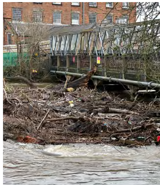
Fig.48 Debris build-up against bridge following during 2024 floods (image – Derby City Council engineers).
