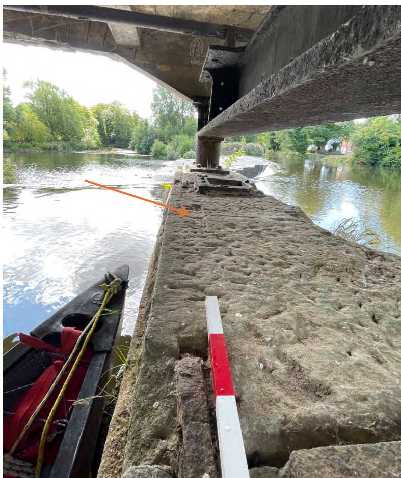
Fig.39 Stone pier with second cast-iron square collar, slightly smaller, approximately 400mm x 400mm. Four corroded bolts to the upper face, one with a surviving threaded nut. Inset timber post with heartwood. Wrought-iron masonry cramps are visible (bottom left of image and top) – 8.8.2025.
