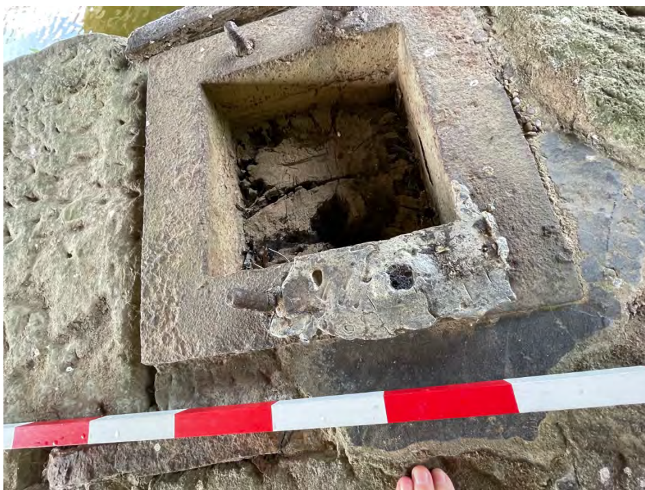
Fig.39 Stone pier with second cast-iron square collar, slightly smaller, approximately 400mm x 400mm. Four corroded bolts to the upper face, one with a surviving threaded nut. Inset timber post with heartwood. Wrought-iron masonry cramps are visible (bottom left of image and top) – 8.8.2025.
