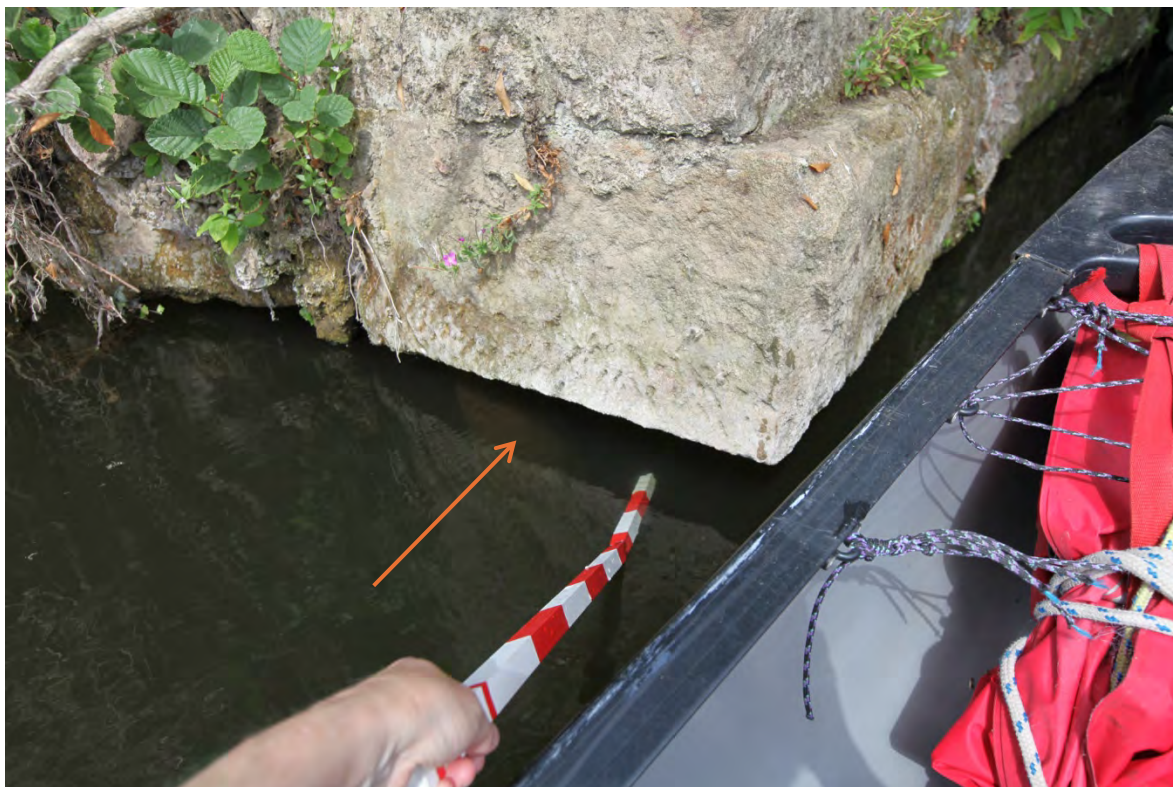
Fig.32 Undercut to right abutment of 1.5 metres, with pile arrowed (8.8.2025).
