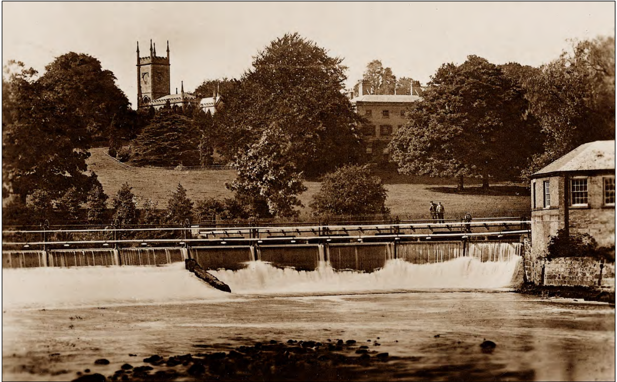
Fig. 7 View of Darley House, the Church and the Canteen (courtesy Adrian Farmer), ca. 1920s. The view shows the weir with its sluice gates lowered and the rack-and-pinion mechanisms and narrow boardwalks in-situ. In the background, the bridge has flat soffits, with broad flat spandrels over the posts, narrow railings, without concrete pillars, and appears to be a concrete precursor to the concrete and rebar bridge of 1934. The cast-iron end-caps can also be clearly seen.
