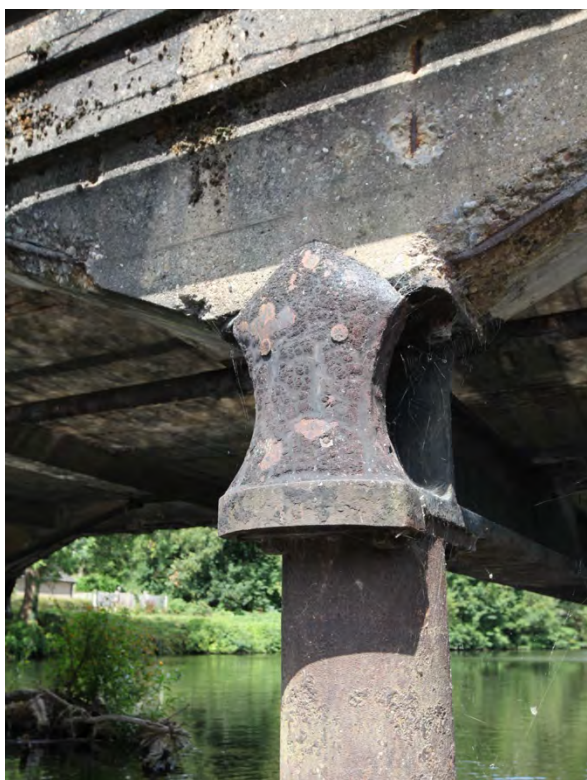
Figs.43 & 44 End caps with visible dowels to upper face (left – plain, right – with 1853 date in the casting) – 8.8.25.
