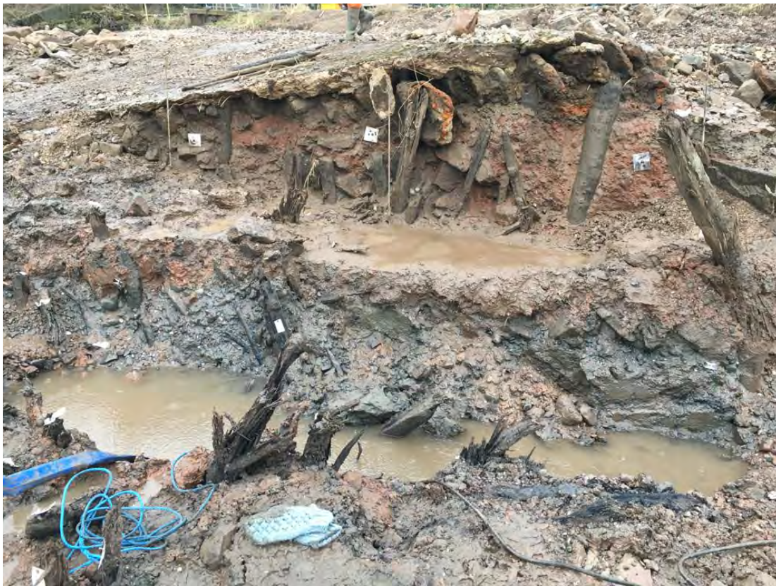
Fig.47 Dovecliffe weir removal. The timber and clay packing of the earlier weir beneath the stone and later concrete cap (YAT).
