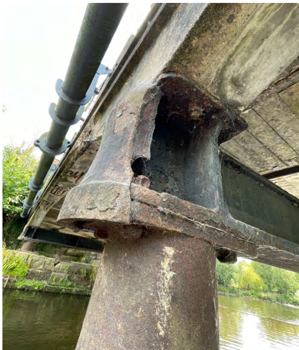
Fig.42 Castings for the beam and post meet with a flat joint which is part covered by the bell-shaped end cap. Here there is some local corrosion which has exposed one of the bolts - 8.8.2025.
