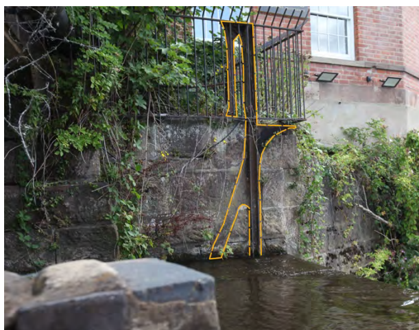
Fig.45 Left bank at the weir crest. Marked in yellow dashes is the casting for sluice gate, rack-and-pinion and grooves for raising the gate within the 'wing wall' - 8.8.2025. The outer spur carried a narrow boardwalk.
