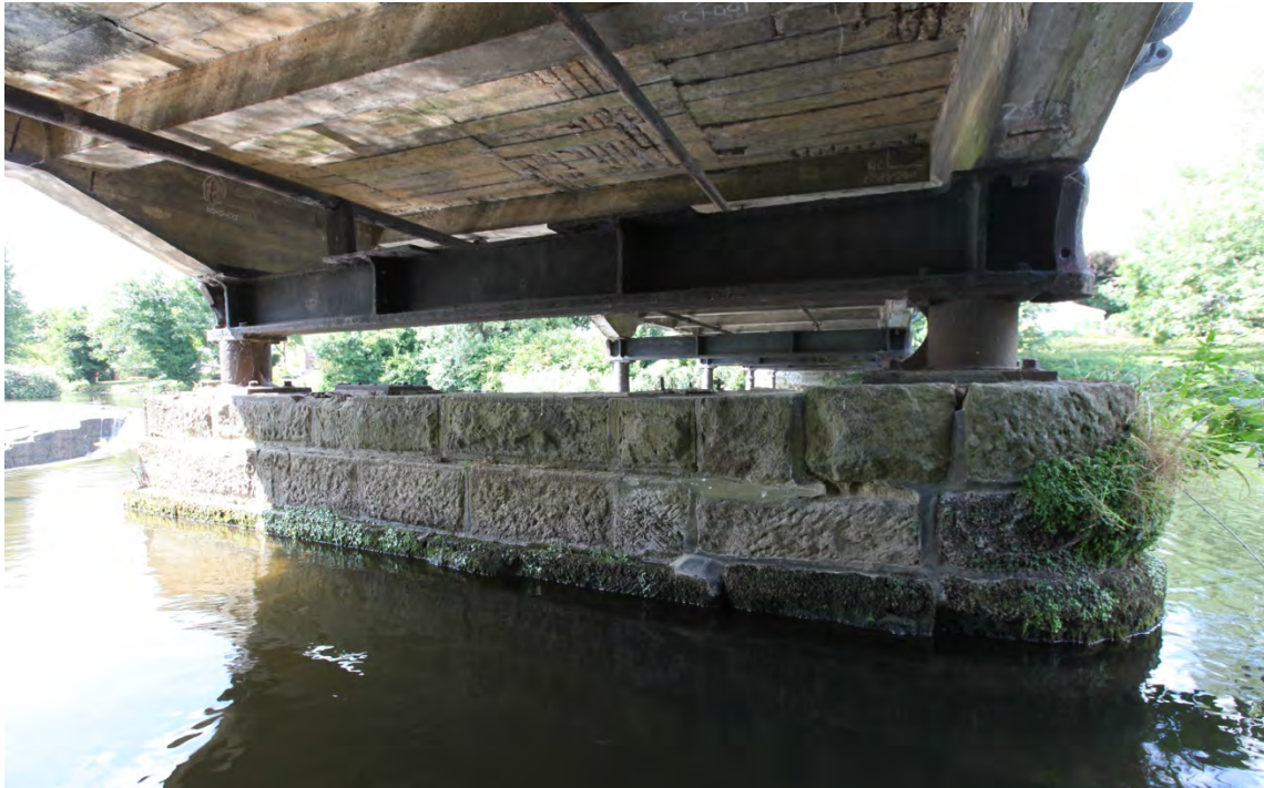
Fig. 37 Stone pier with short cast-iron posts, transverse cast I-beam, and rounded cutwater - 2025
