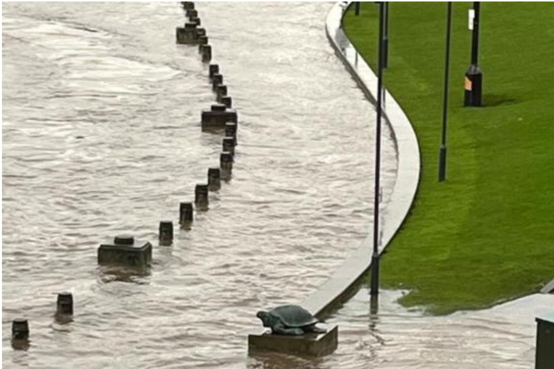
Flood walls at the River Gardens on 21 October 2023
