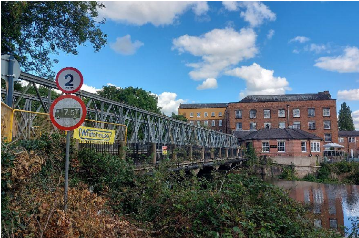
The temporary Walter's Walkway at Darley Abbey
